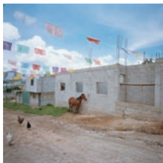
Page 15: New houses are almost always built with cinder blocks, Mirador, 2007.
